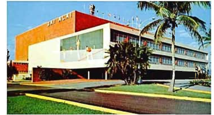
ORIGINAL JAI ALAI FACILITY IN 1978
